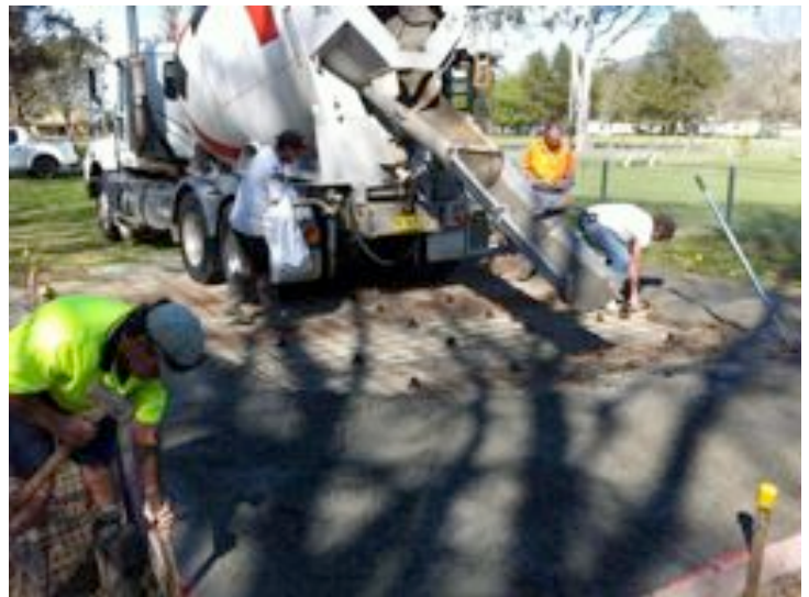
Exercise equipment slab preparation and pour.
